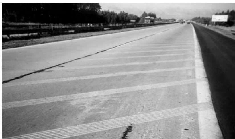
**Figure 1: Grooved drain lines on a concrete motorway pavement surface**
