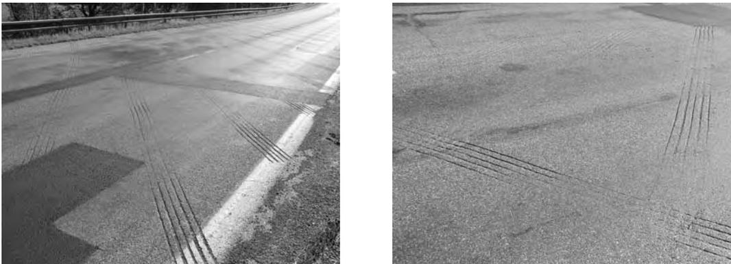
**Figure 3: Grooved drainage lines on I/34 highway, exploited and deteriorated treatment**
